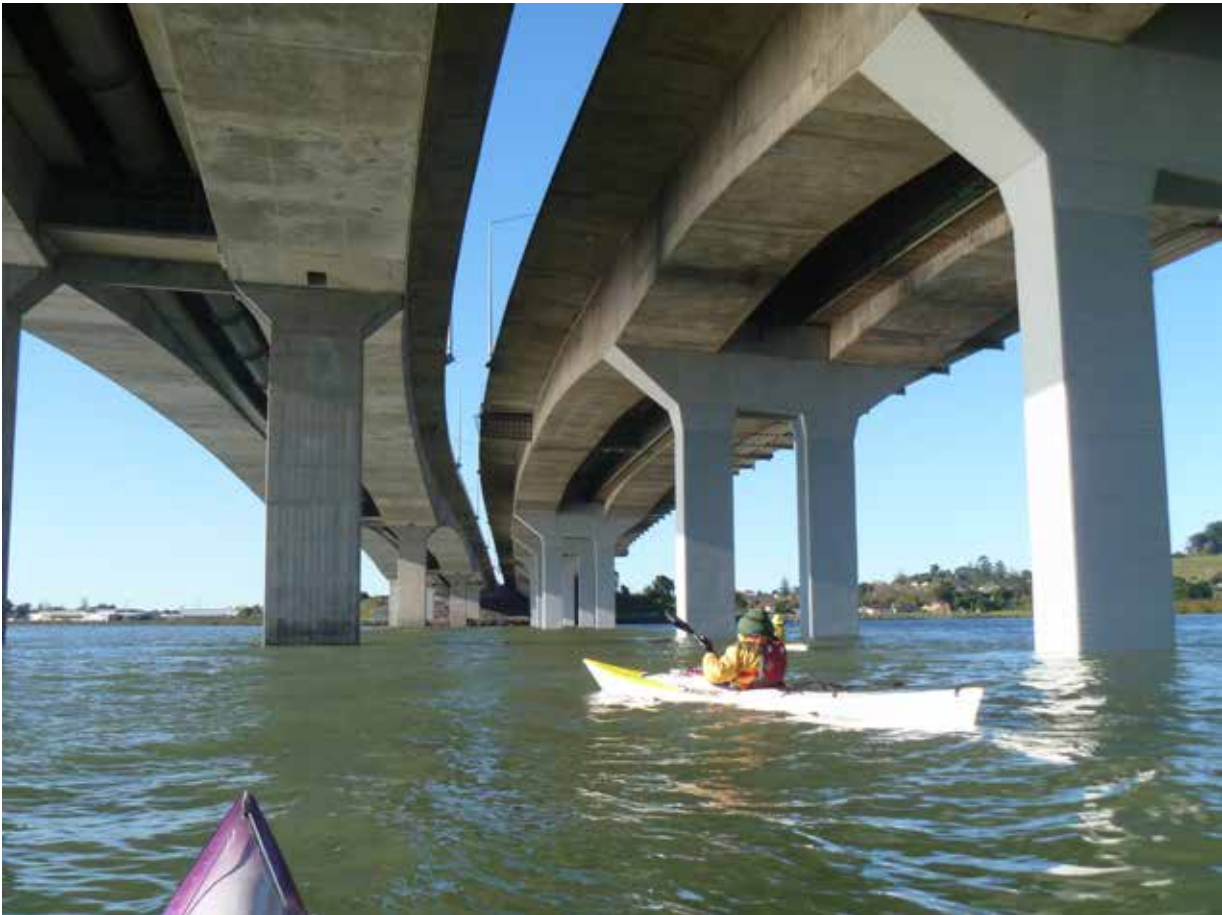
Early morning kayakers doing the Mangere Bridge circuit.
