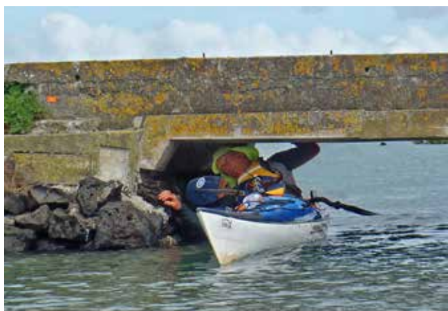
A tight fit for Mike Randall beneath the causeway bridge.
