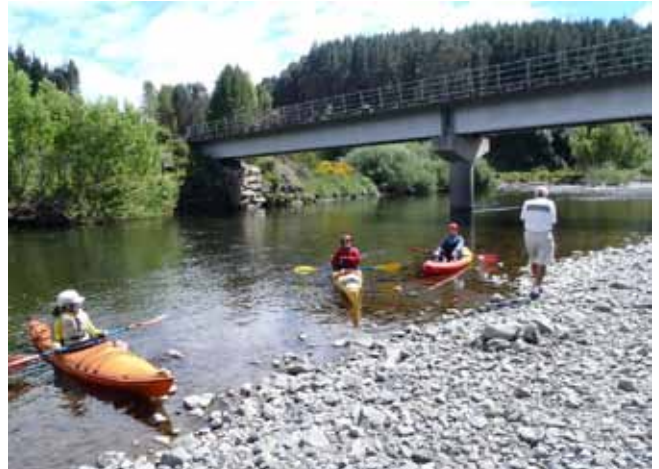
Pukaututu Road bridge
