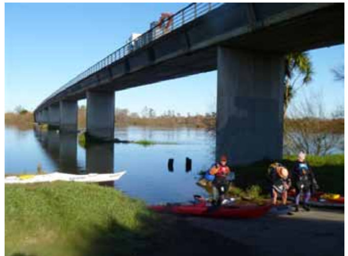
▼ Rangiriri bridge ramp and time for a cuppa.
