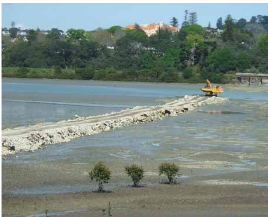
Causeway pipeline removal Purewa Inlet.
