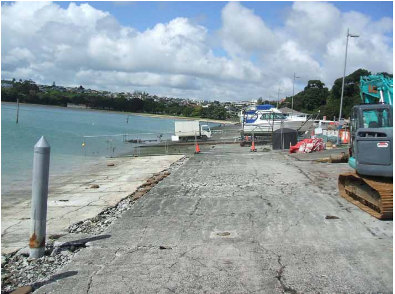
WORK IN PROGRESS. The Okahu Bay ramp upgrade has commenced.
