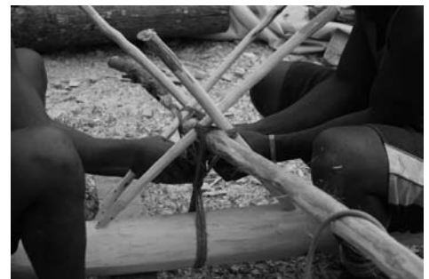
Stitching and lashing the components together
