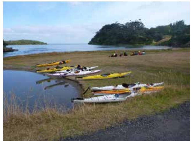
The small bridge at Gardiner Gap was strengthened some years back. Substantial laminated beams were installed, diminishing clearances for kayakers passing below. On some big tides passage is restricted. These kayakers enjoy a picnic near the bridge waiting for the tide. The grassy area was once a summer campground.
