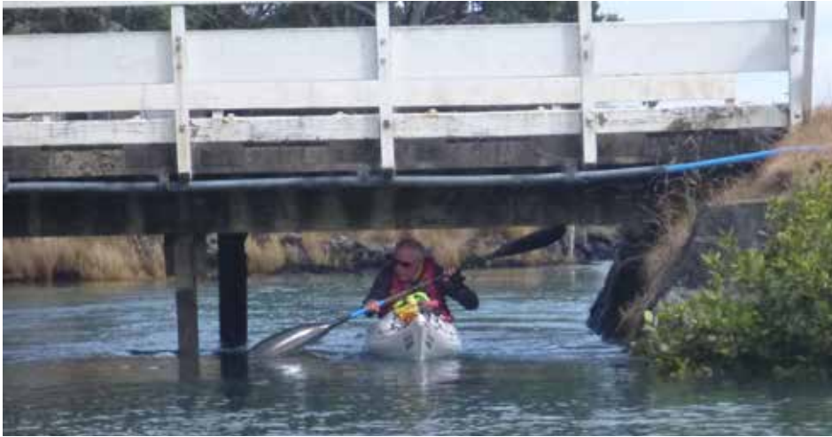
Club kayaker Ian Smeeton negotiates the causeway bridge at Gardiner Gap. This was almost an hour after peak tide. The bridge support strut on the outer left clearly shows the high tide mark.
