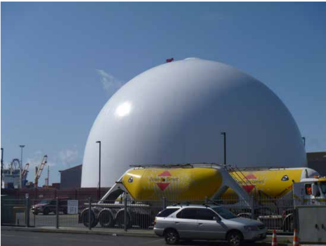
Almost in the blink of an eye, one of these popped up on the waterfront opposite Vector Arena. It's a new cement silo with a capacity of 30,000 tonnes. Nearby are two rectangular shaped silos. Somehow you get the feeling that the waterfront might need another one of the curved silos to balance things out.
