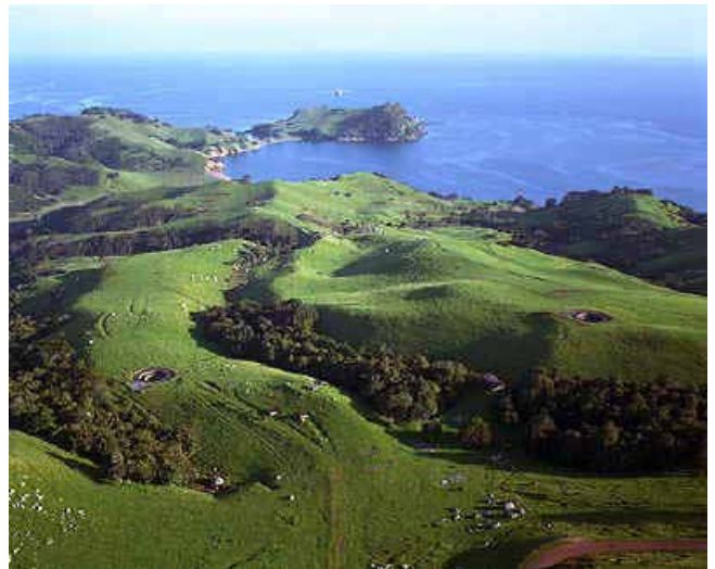
An aerial view of the present day Stony Batter with two of the circular gun emplacements visible. Hooks Bay and Thumb Point are beyond.
