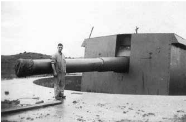
One of the big 9.2 inch Stony Batter guns. They were only fired a couple of times for testing.
