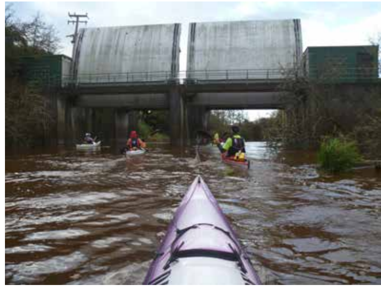
These floodgates, located at the very lower extremities of the Whangamarino River, act as guardians for the wet-lands beyond. The paddlers are all looking a bit anxious because some wag has just advised them to be wary of their rapid guillotine like action during closure.
